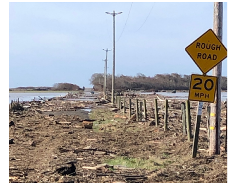
Flood debris closing Cannibal Island Road
